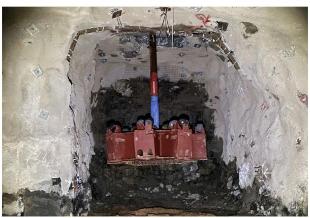
Figure 5 - Reamer installed and ready to commence back-reaming the 4.5m diameter return air raise
