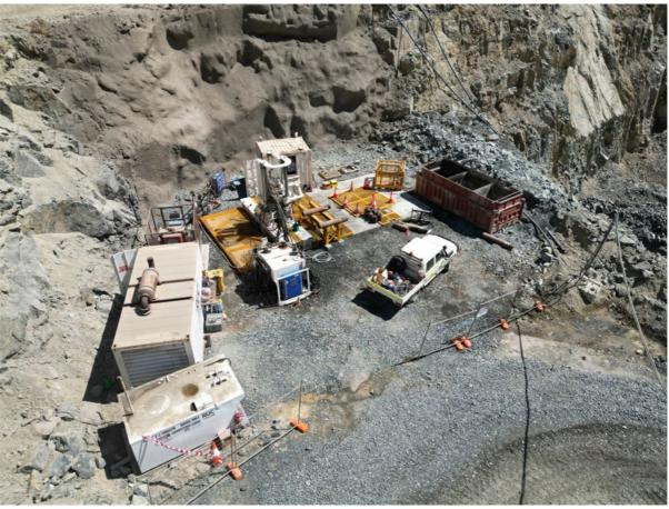
Figure 4 - View of the raisebore machine setting up to commence back-reaming the primary return air raise
